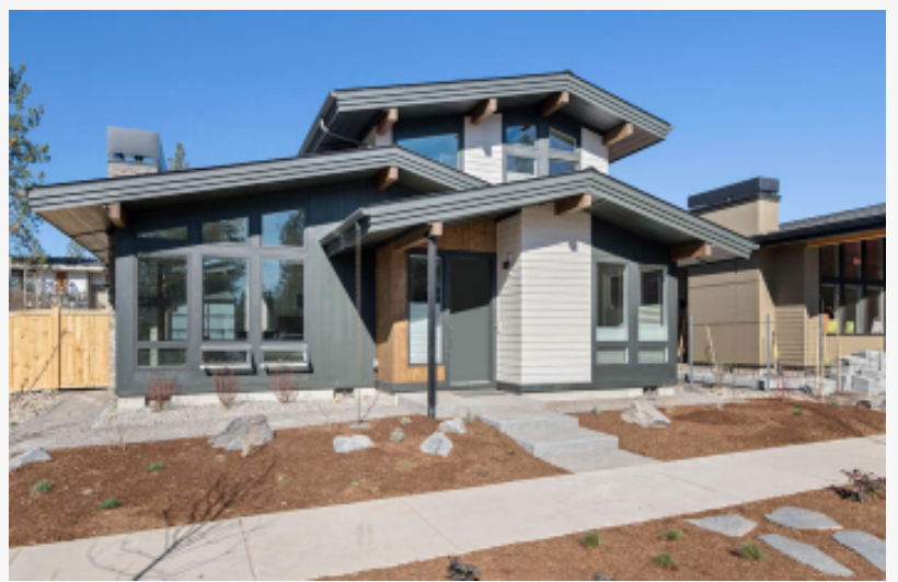
JD Neel Construction home in Bend, Oregon's Discovery West
